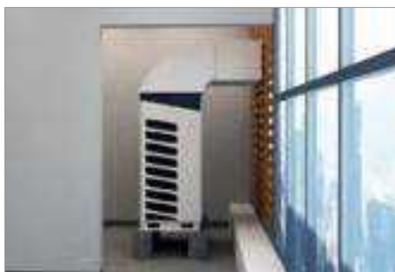
Installation du gainage
